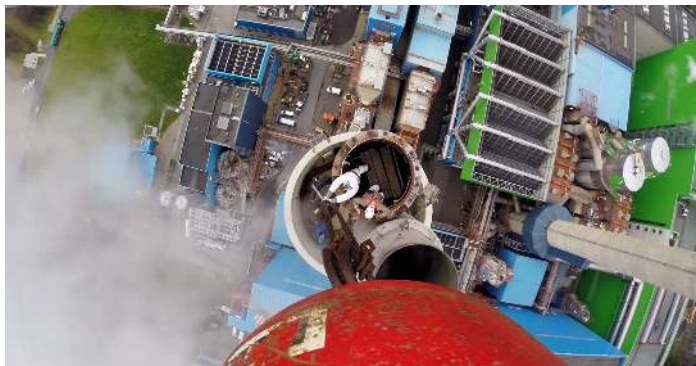
TECHNICIANS INSIDE THE FLUE MOUTH · LIVE PLANT
